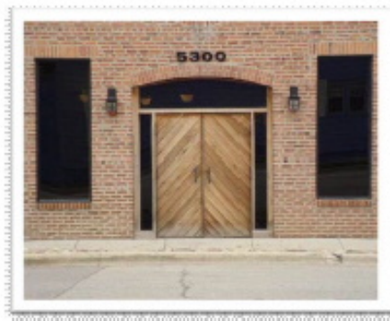
Figure 18: Discouraged Entryway - Opaque windows, and windows that do not make up the majority of the storefront give the appearance of a residential entryway rather than an entryway of a commercial building.
