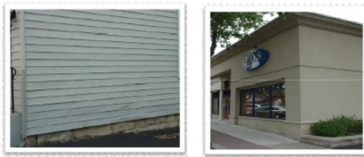
Figure 7 Discouraged Materials: Use of vinyl and aluminum siding, and EIFS as a primary material is discouraged.
