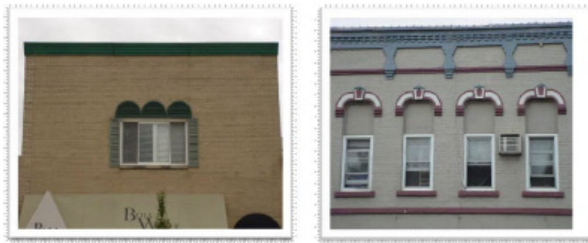
Figure 13: Discouraged Windows - Windows that are both not to scale with the façade or the traditional window openings.
