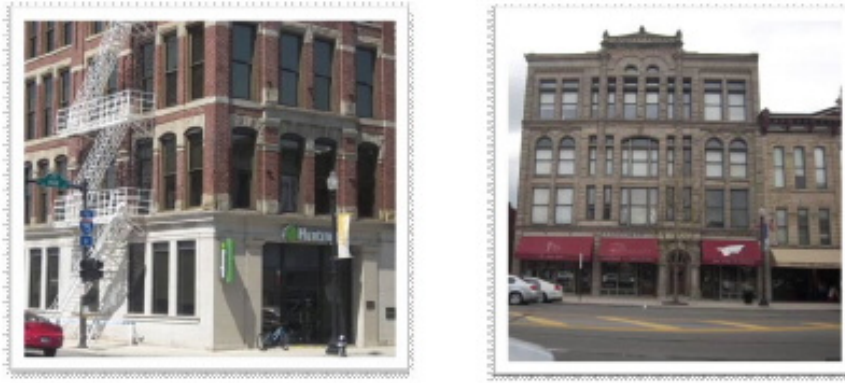
Figure 6 Appropriate Building Materials: Good use of brick, stone, and canvas awnings.
