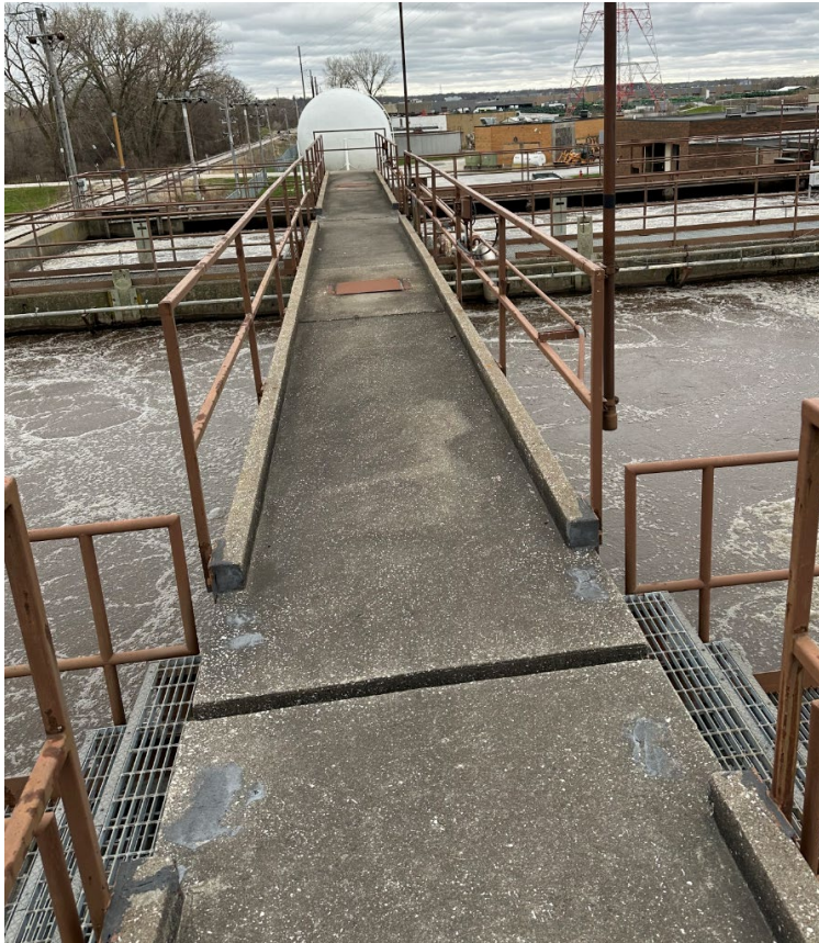
Aeration Tank Walkways and Handrails
