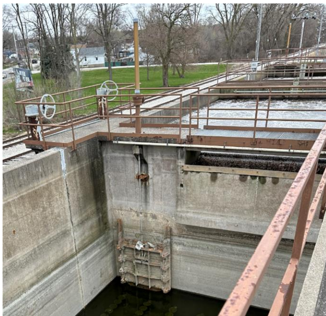
Figure 8 Existing Sluice Gate Between Aeration Tank Nos. 2 and 3
