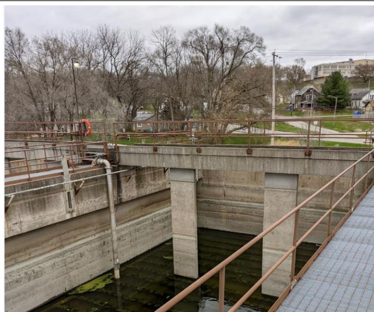
Figure 9 Aeration Tank Precast Bridges
